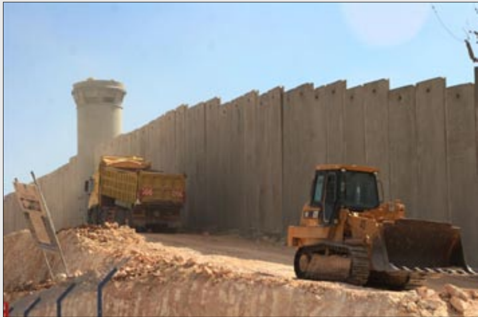
Constructing the Wall around Jerusalem with Caterpillar equipment. © Anne Paquier.
